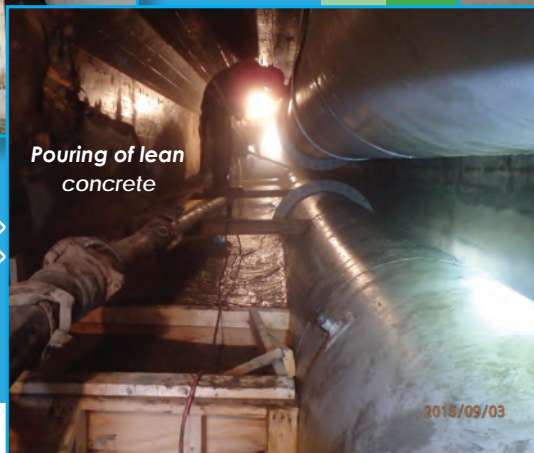
12" conduit for electrical and raw water taps
