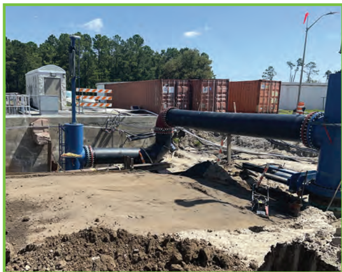
Line stop piping for LPRO tie in
